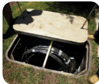
A construction pit in Kiama, New South Wales.
