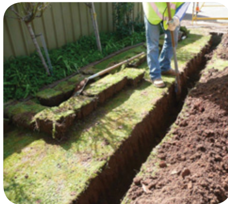
Digging a residential trench to lay fibre optic cable.
