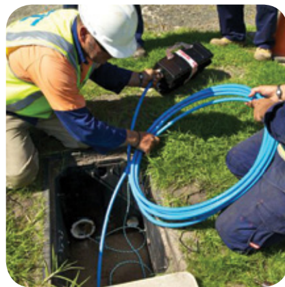
Underground fibre hauling in Kiama, New South Wales.
