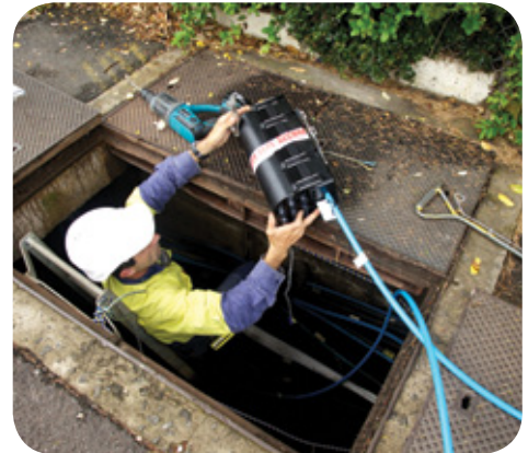
Use of an existing pit in Brunswick, Victoria, a First Release Site.
