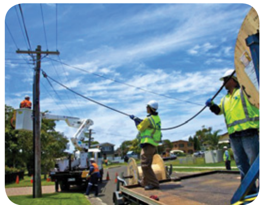
Aerial construction in Kiama, New South Wales.
