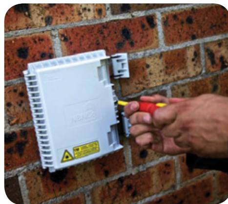
Typical Premises Connection Device used in Kiama, New South Wales, a First Release Site.
