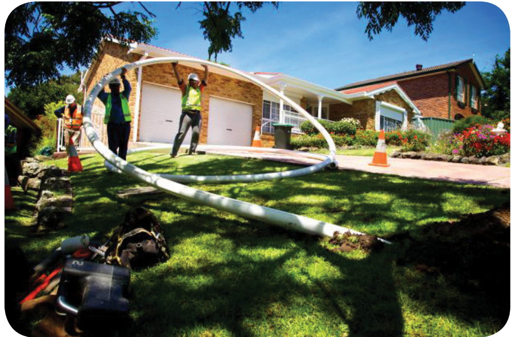
Laying pipe in Kiama, New South Wales.
